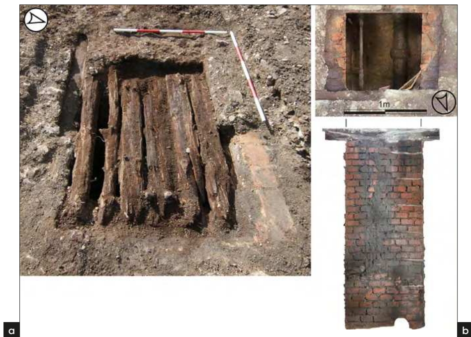
Fig. 10. Revision shaft at the camp sewerage close to the kitchen building: (a) temporary covering of the shaft with secondary used beams that were poured with a thin cement mixture, which is already removed on the field photograph (photograph by D. Pilař); (b) plan and southern profile of the shaft.
